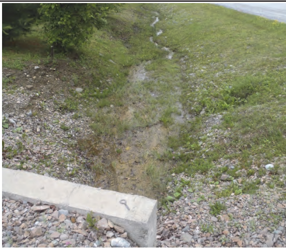
Photo 1. Erosion around culvert header.
