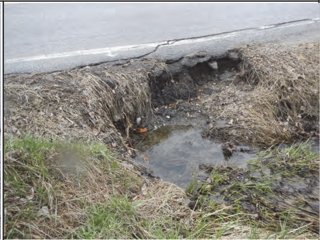
Photo 2. Pavement erosion
