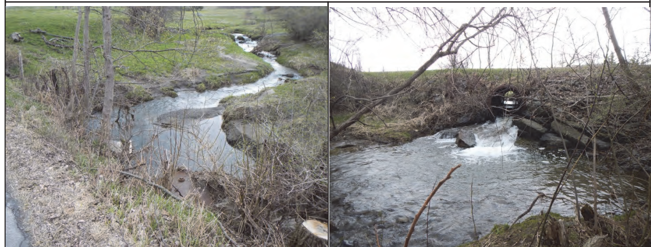
Photo 1. Upstream banks are unstable and meandering Photo 2. Culvert outlet and scour pool
