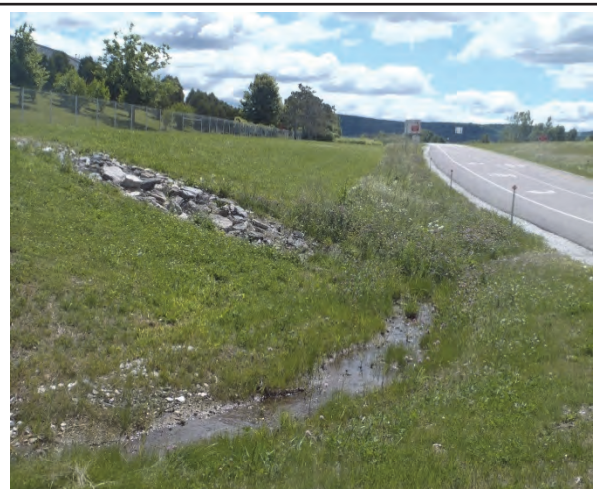
Photo 2. Intersection of Route 207 and I-89 off ramp
