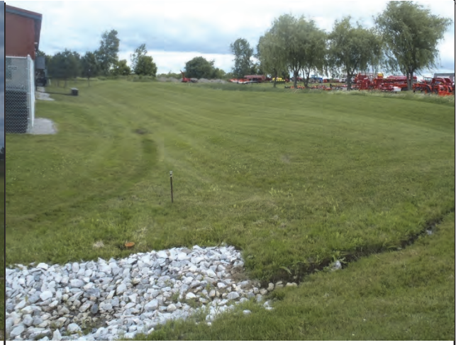
Photo 2. Eroding swale near F.W. Webb
