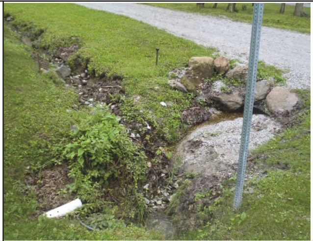
Photo 2. Plugged culvert
