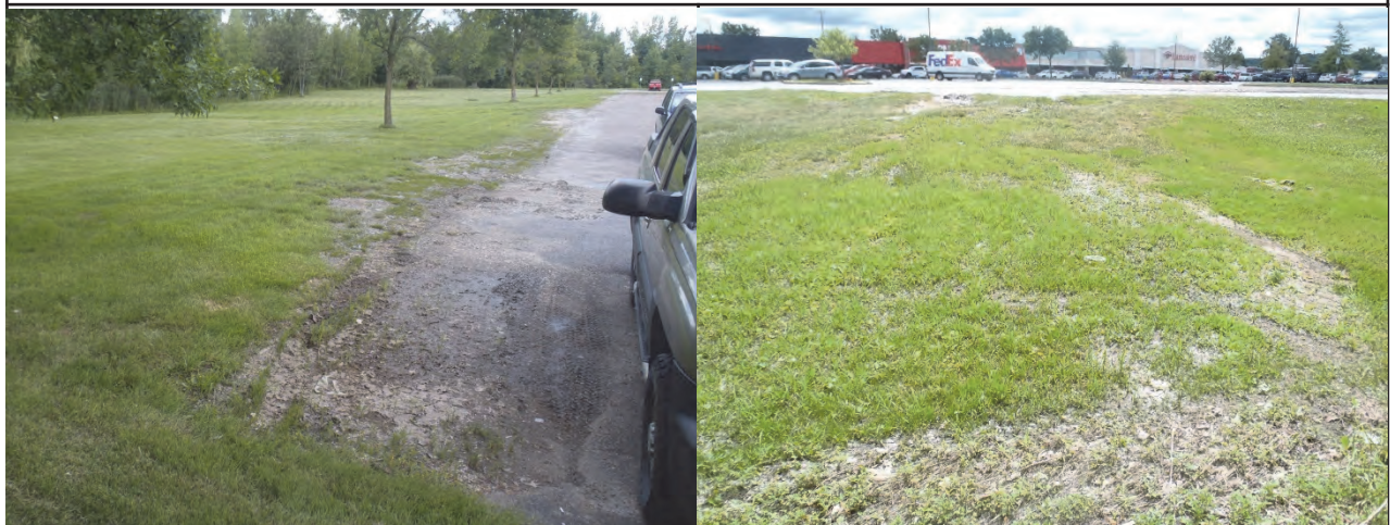
Photo 1. Evidence of stormwater draining off wet edge of parking area
