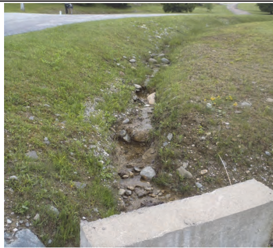
Photo 2. Erosion upstream of culvert header.
