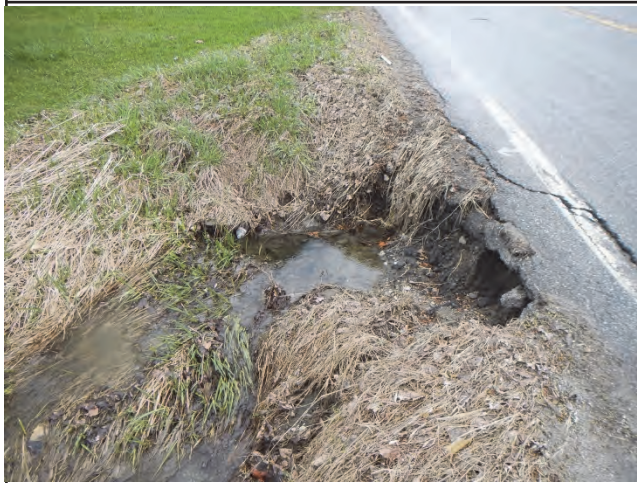
Photo 1. Pavement erosion at culvert outlet
