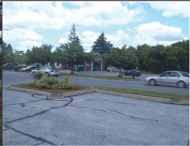
Photo 2. Example of island used to separate parking areas from travel lanes.
