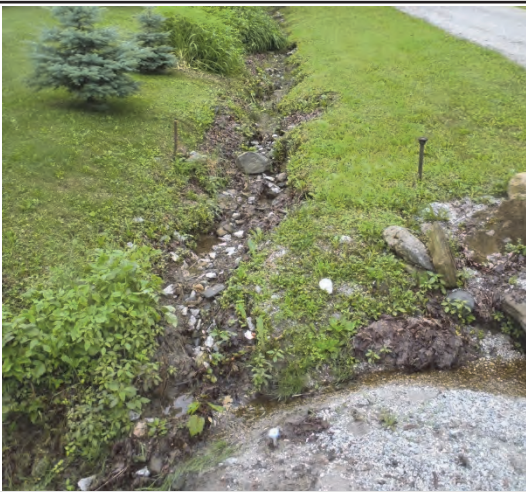
Photo 1. Actively eroding ditch.
