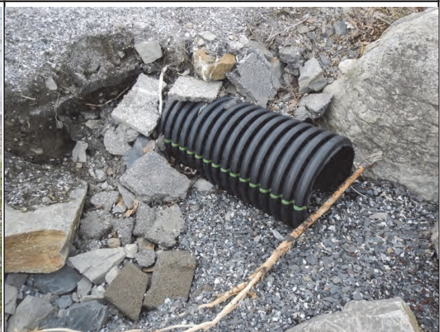
Photo 2. Erosion around outlet
