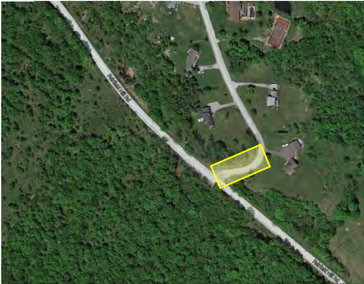
Figure 7. Area of active erosion near the intersection of Lakemont Drive at Fairfield Hill Road.
