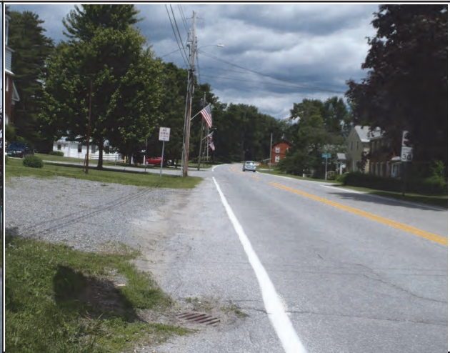
Photo 2. Catch basin that receives runoff from Town Hall
