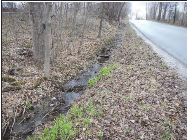
Photo 1. Incised ditch bottom Photo 2. Ditch path to Stevens Brook
