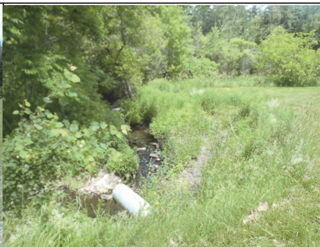
Photo 2. Evidence of bank slumping and direct stormwater discharges.
