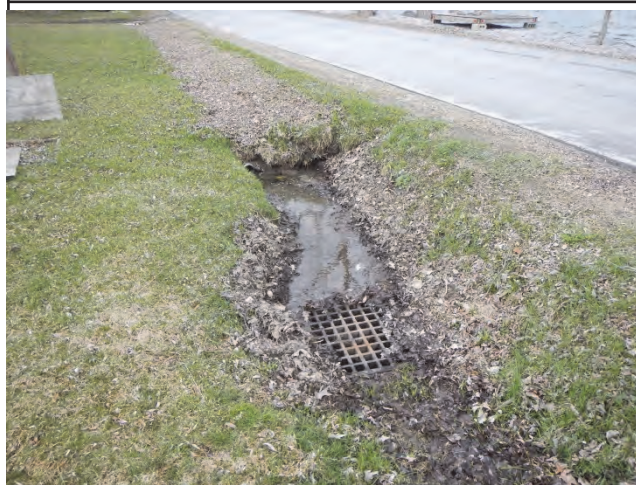
Photo 1. Erosion near catch basin
