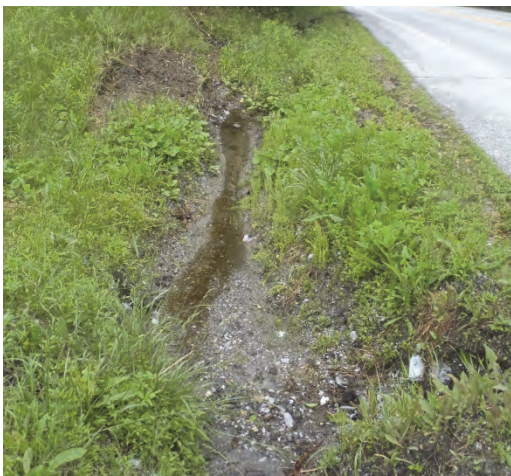
Photo 1. Evidence of sediment from Lakemont Drive being deposited in ditch along Route 36
